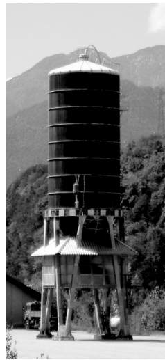
(e) Salt storage with control room, Italy
