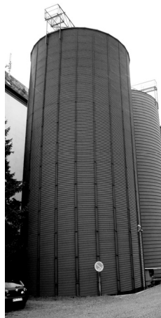
(b) Corrugated steel storage, Germany
